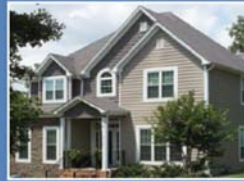
Roof, Siding, Windows & Stone Installation
