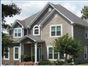
Roof, Siding, Windows & Stone Installation
