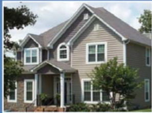
Roof, Siding, Windows & Stone Installation
